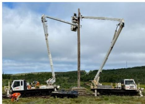
Single pole construction on transmission line 94L.
